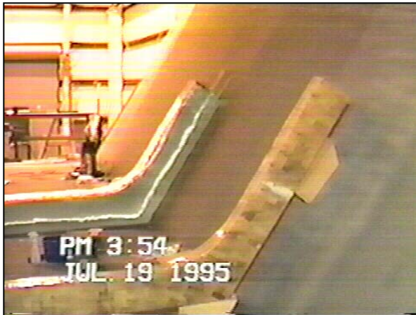
Ring Girder Installation
