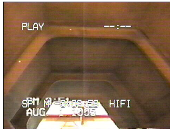
Ring Girders Laminated In-Place
