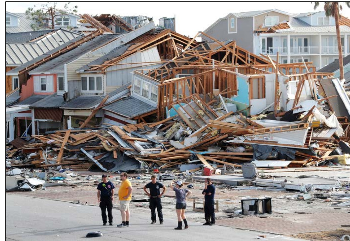
Damage from Hurricane Michael, Florida Panhandle, Oct 2018
