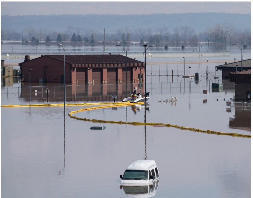
Offutt Air Force Base - One-third of the installation was flooded, and the containment boom was a precautionary measure for possible fuel leaks. (US Air Force photo by Delanie Stafford)
