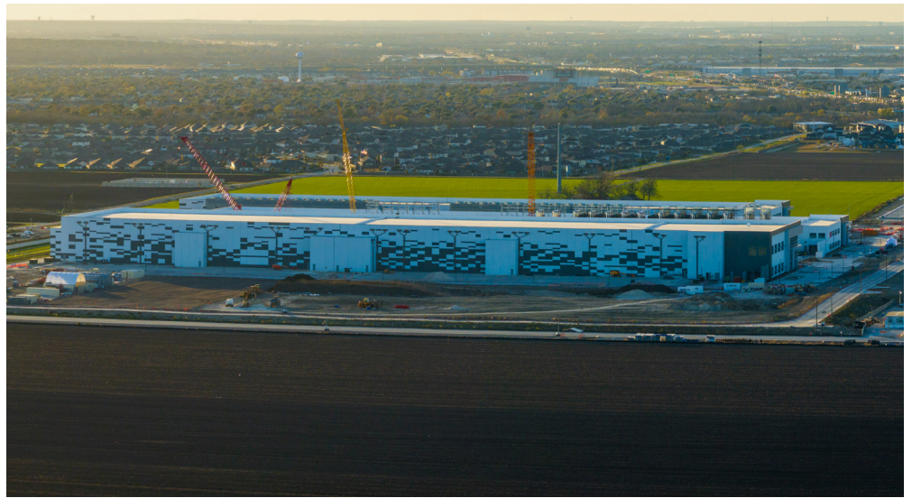
The Skybox Prologis PowerCampus Austin, located in Hutto, TX, is a 160-acre hyperscale data center campus designed specifically for high-density AI and cloud computing workloads.
