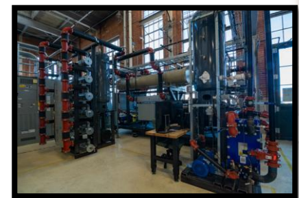
300 kWth heat activated cooling system (TCCS)
